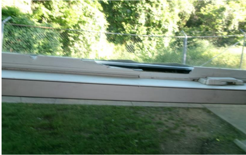
*broken window framing unit 145*
